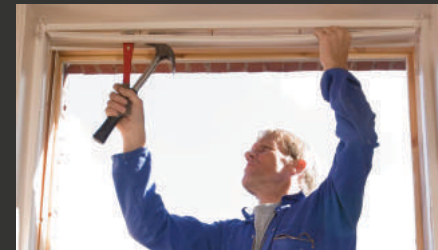
Remove mitred bead from around frame
