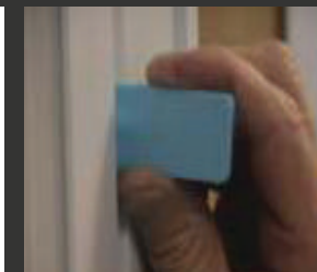
Installation Packers
