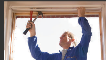
Remove mitred bead from around frame
